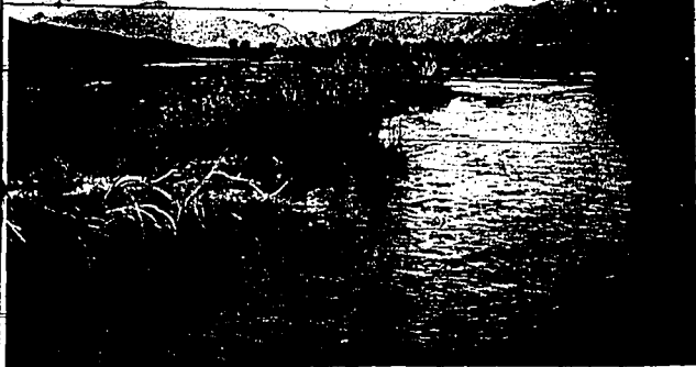
FLOOD CONTROL WORK on Big Lost River, carried out under the direction of the Corps of Army Engineers. In the past month, has resulted in rechanneling of 16 per cent of the stream. The work was done on 11 sites, covering about 8.1 miles of the 51-mile length. Three sites were completed above Mackay Reservoir with the other 11 from the dam to Arco.
