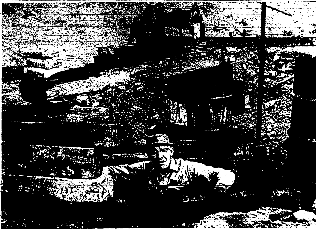
THIS LOOKS TO BE a fairly primitive operation, but Al Smith, leaning out of the hole he dug with pick and shovel, says it's a small but steady producing oil well. With his digging
