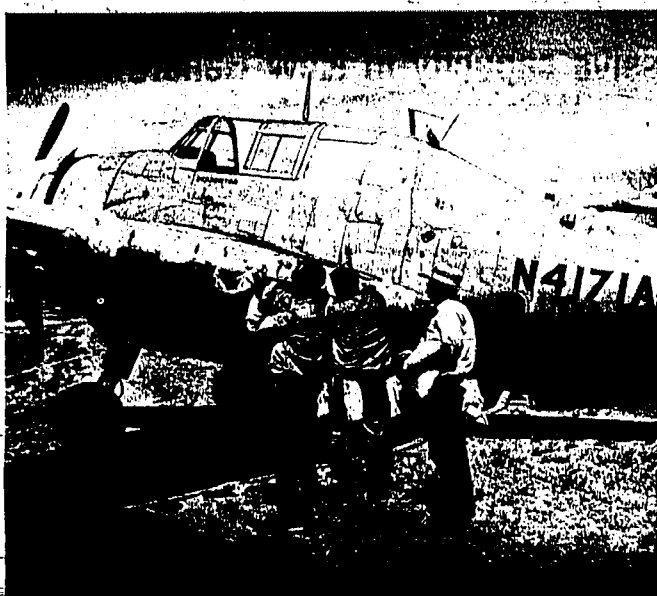
WORLD WAR II bomber, one of many which has been refitted as a spray plane, is checked by forest workers to make sure it sprays at the proper rate of 13 ounces to the acre. These planes are flown low and in sometimes dangerous areas by expert pilots. (U. S. Forest Service photo)
