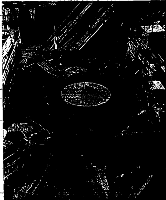
COMPLEX ASSEMBLY of three generating units proceeds in depths of future powerhouse. Welders at center are completing fabrication of small-like steel tube that will distribute water around wheel on one of the unit's turbines. (Idaho Power photo)
