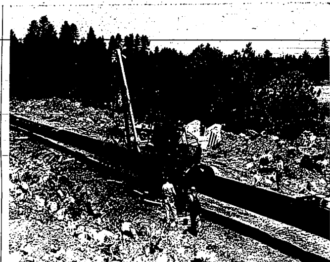
NATURAL GAS on its way to Idaho. This is a portion of the 1,500-mile long 26-inch ribbon of steel which transports natural gas from New Mexico and Canada to Southern Idaho. This pipeline makes more energy available to Southern Idaho than in the energy output of six Hoover Dams. The pipeline has been in Southern Idaho for 10 years.
