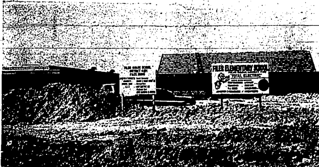
ONE OF THE many new buildings taking shape in Magic Valley under the guidance of area construction firms and general contractors is the new Filser school. The modern school, designed to take care of any educational technique that may come along in the next 30 years is being built by Neilson and Miller Construction Co. (Times-News photo)
