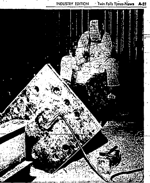
HEAVY STEEL BEAMS like the one above are just routine items in the list of fabrication jobs handled by K and T Steel Corp., Twin Falls. Here a welder fits a moving 'choker' while he welds a seam in the heavy steel beam. Formerly Self's Manufacturing Co., the firm now specializes in heavy steel construction. (Times-News photo)
