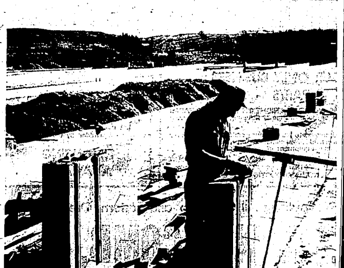
SMOOTHING THE CONCRETE on top of one of the walls of fish ponds at the new Clear Springs Trout Co., Inc. hatchery, north of Buhl, is Ted Eastman, manager. The hatchery is nestled between Clear Lakes and the Snake River canyon. Some 10 ponds have already been built, and when completed, the hatchery will have 20 ponds. (Times-News photo)
