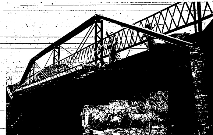
SANDBLASTING OPERATIONS are under way on the 60-year old Perrine Bridge in the Snake River Canyon north of Twin Falls. Purchased by the city of Twin Falls, the bridge is being prepared for renovation and painting for its future role. It will support a 36-inch steel water main across Snake River as part of the new city water system. Operating sandblasting equipment is Max Stuart of Stuart Bros. Contracting Contractors. (Times-News photo)
