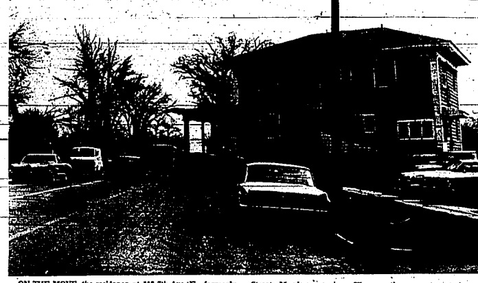
ON THE MOVE, the residence at 116 7th Ave. E., formerly owned by Ernest Wills, Twin Falls, edged out onto Shoshone Street Monday morning. The one-time apartment house will be placed on foundations on the canyon rim northwest of Twin Falls by the Gun Club. (Times-News photo)
