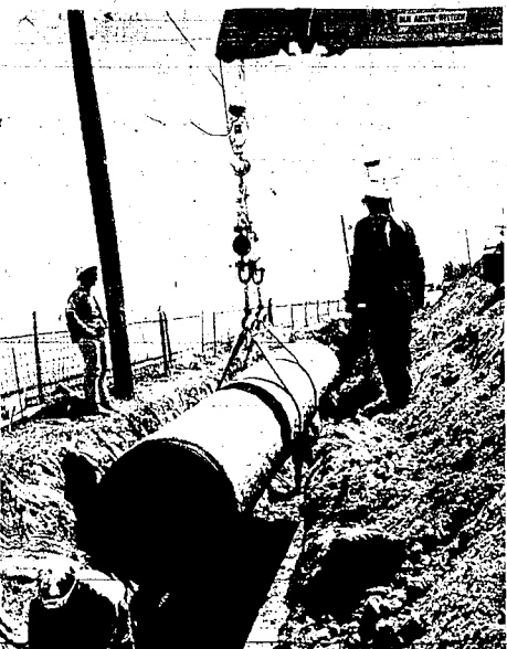
EQUIPMENT AND CREWS OF Kloepper Construction Co., Logan, Utah, swing a giant section of 36-inch pipe into trench on Washington Street North, line of three major contractors working on the Twin Falls water improvement project. Kloepper is currently installing the line from the upper rim of Snake River Canyon to the main city distribution system. (Times-News photo)
