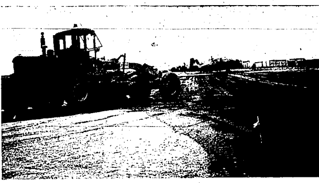
FOOTBALL FIELD-SIZED parking area for fire-fighting airplanes is not under construction at Twin Falls Municipal Airport. Here, City Street Department crews grade the area as they get ready for final work on the project. The area needs to be finished by the time the fire season begins, about the first of July. The area is expected to relieve congestion caused by the large number of planes, such as the one in the background, using the area. (Times-News photo)
