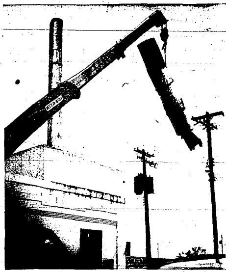
STACK COMES DOWN from the roof of Toy National Laundry and Dry Cleaners building via a large crane Tuesday afternoon. Bill Povel, manager, said the top 10 feet of the 60-foot stack blew off during a heavy storm last fall and had remained atop the building since then. He said the 30-inch pipe had been weakened by rust, causing it to topple in the wind. The top of the remaining stack was trimmed, he said, because such a long stack has not been necessary since the firm converted to gas. (Times-News photo)
