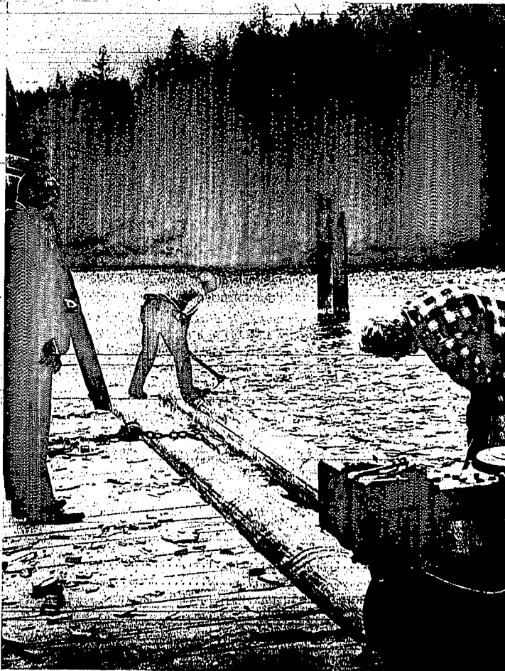
INSPECTS work on boat docks on Buttonhook Bay at Farragut State Park.
