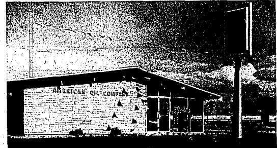
Pictured here is the modern new office, administration building and air conditioned meeting room that will allow us to serve many of the needs of this area.
