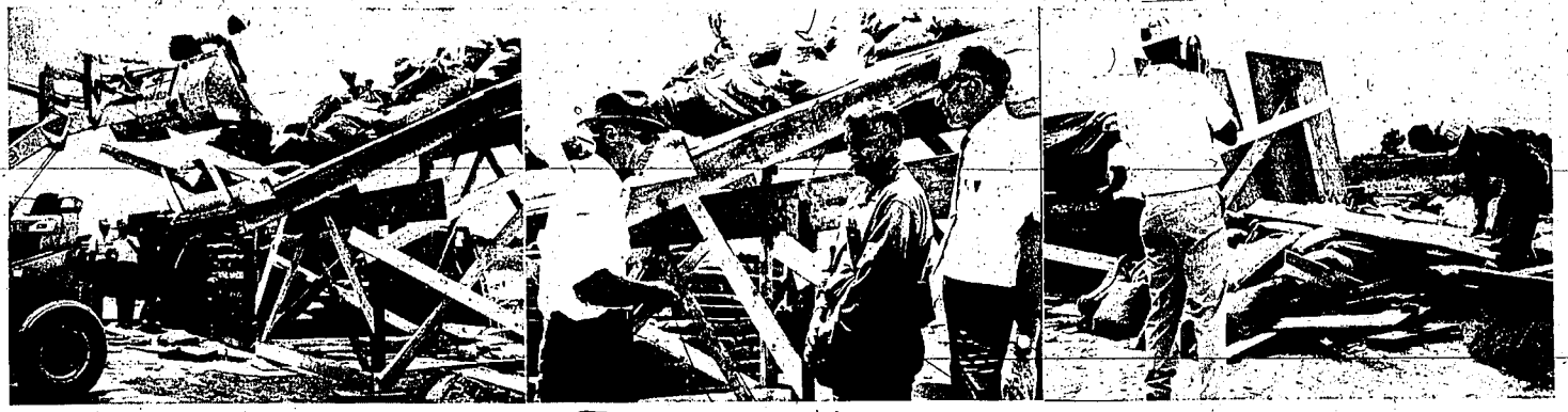
JUST HOW MUCH weight will shoring support safely is the object of tests conducted at the site of the Twin Falls reservoir. At left, Don Hillman, Crom Prestressing-Inc.
