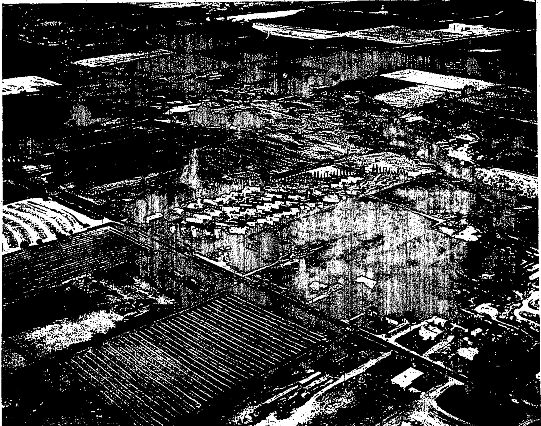
SHOWING MOBILE home living in Magic Valley in this aerial view of the Grandview Trailer Courts located west of the city of Twin Falls in a farming district. Living in these "homes on wheels" is becoming more popular throughout the United States. Twin Falls offers several parks for trailer owners traveling through the city as people add a trailer unit
