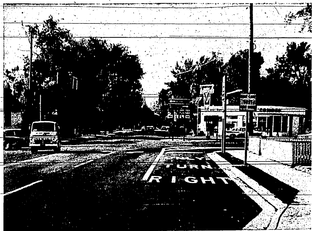
NEW "RIGHT TURN ONLY" lane at the Five-Points-North-Blue-Lakes-Blvd. N., and Addison Avenue to accomplish the additional lane. State workers have just completed painting turn arrows and other traffic directions on the new intersection. City and state crews cooperated in the widening of both
