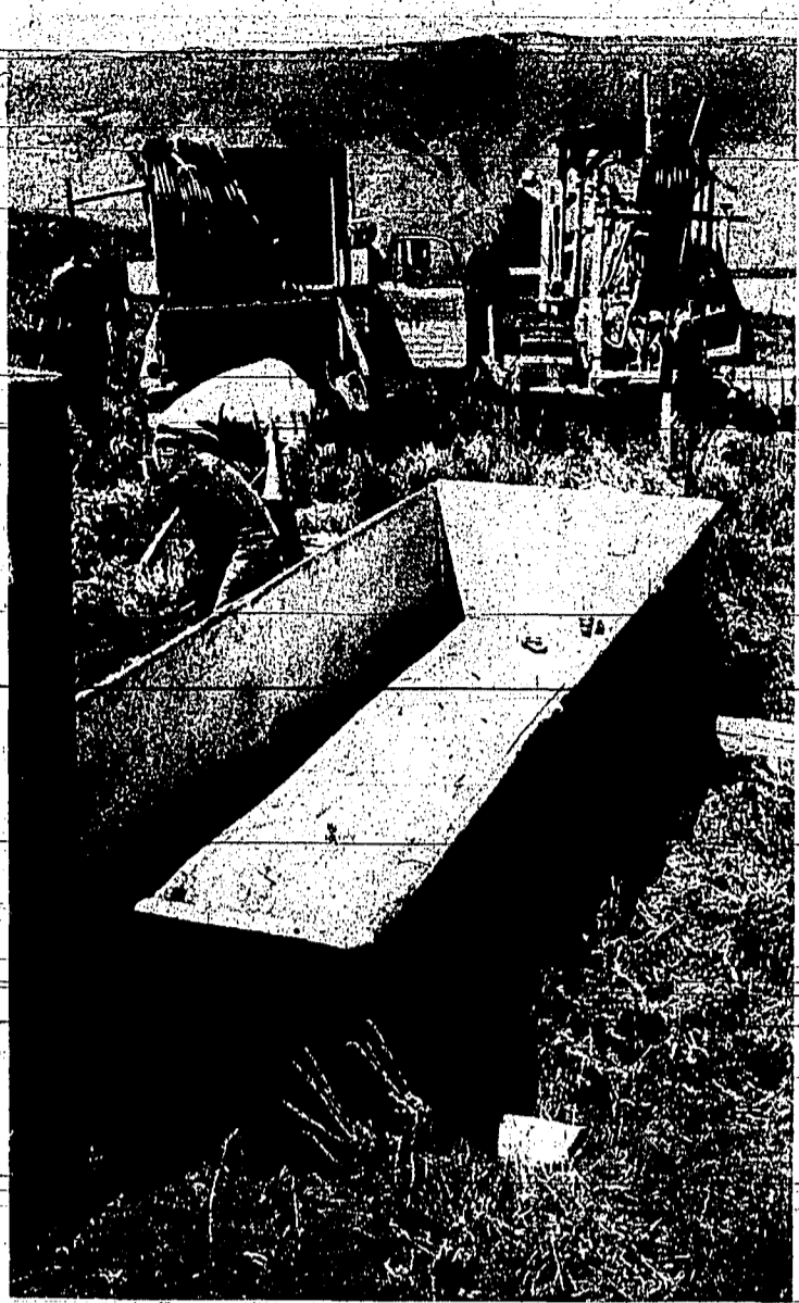
BLM RANGE CREW from Salmon is shown installing a water trough for livestock grazing on the South Carmen Creek unit. Plastic pipe is laid just below surface of ground by machine in background. Water is piped from nearby spring.
