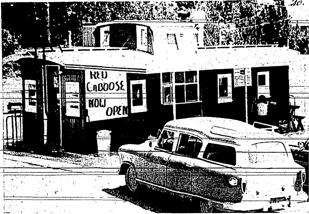
WORK IS NEARING completion on Kimberly's newest eating establishment, the Red Caboose, owned by Mr. and Mrs. Edward Thompson. The caboose, purchased from the railroad firm, had been retired after 60 years of service in the West
