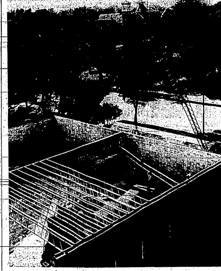
ROOF TRUSSES are being swung into position along the south half of the Twin Falls County Courthouse judicial annex, as seen from the roof of the courthouse proper. Within a week, building officials say, they hope to have the entire roof over the structure. It is now approximately 30 per cent completed with Oct. 1 as the hoped for completion date.
