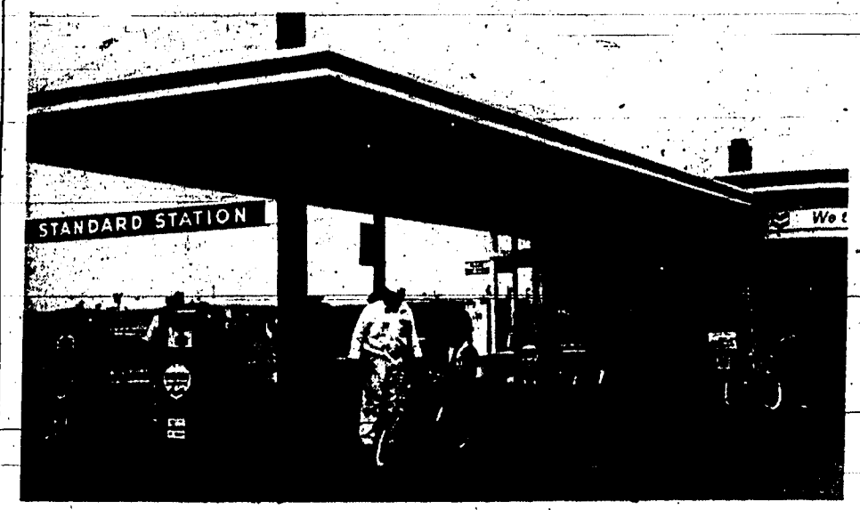
STANDARD SERVICE STATION, the first building in the Lynwood Shopping Center of Twin Falls, opened in 1956.
