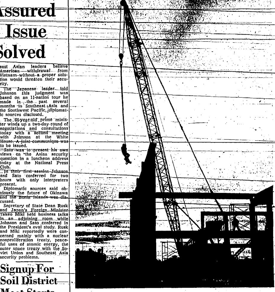
HE FLIES THROUGH the air with the greatest of ease... as prestressed concrete T's are dropped into place on the College of Southern Idaho academic building. The worker on the end of the cable has just helped place one of the huge T's and is riding the cable down to the truck to pick up another T. Work on the campus project is progressing on schedule and brick work has begun on the two-story academic building.
