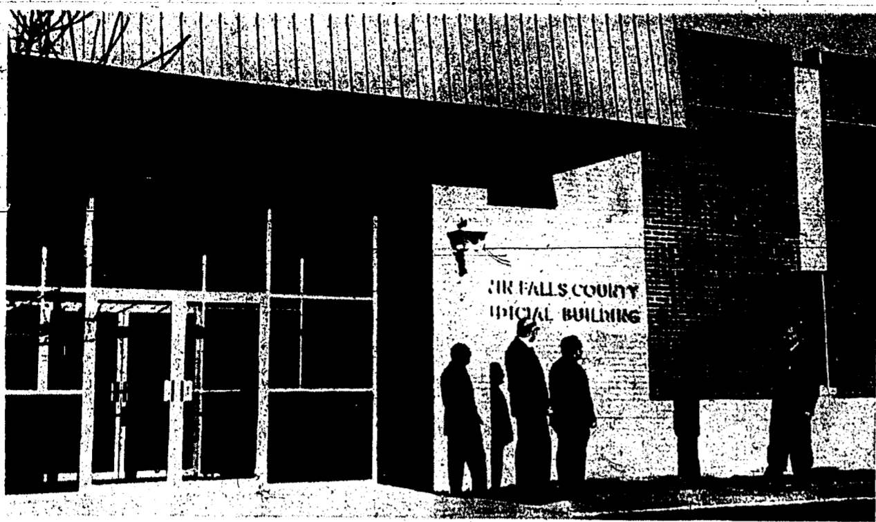
LETTERING AT THE main entrance of the new Twin Falls County judicial building is inspected by, from left, Judge James M. Cunningham, County Commissioner William Chancey and Judge Theron Ward. The building has been completed at a cost of approximately $140,000 despite a law suit brought by general contractors of the area. A State Supreme Court decision on an appeal by the contractors is still pending.
