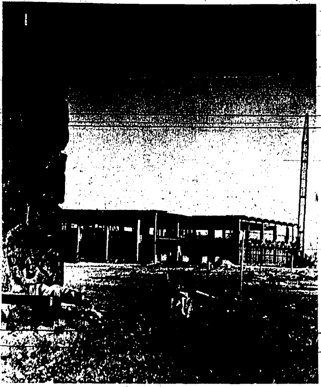
FRAMED BY A PORTION of one of the heating and cooling complexes on the College of Southern Idaho campus is the academic building, one of three major structures under construction. The heating and cooling complexes have been partially faced with native lava rock and are designed to include bulletin board and conversational areas, masking their functional design. Besides the academic building and the heating and cooling complexes, a fine arts center and maintenance building are being constructed. The buildings included in Phase I are scheduled for occupancy this fall.
