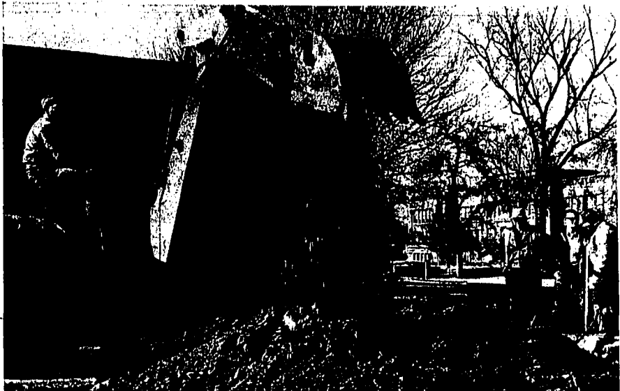
WARM WEATHER and construction go together. Dirt is being removed here to make way for the new addition to the Twin Falls Clinic and Hospital. Construction is expected to be finished by winter. The two-story addition will provide space
