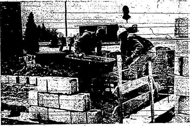
WORK IS PROGRESSING on a 33- by 65-foot addition that will increase the Mountain View Nursing Home, Kimberly, to its rated capacity. This is one of several additions to nursing home facilities now being constructed or in the planning stages.
