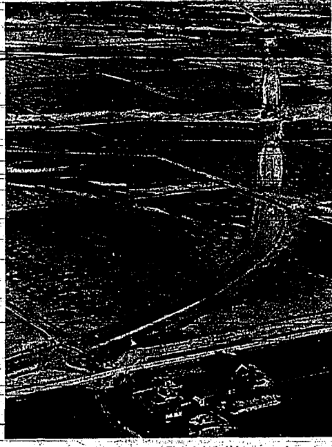
CUTTING PATH through farmland north of Kimberly is the highway now under construction connecting U.S. Highway 30 and Hansen Bridge. This Times-News aerial photo shows the path cut through the farm land and the Hansen Bridge and Snake River Canyon. The farm in the foreground is located about one-half mile east of the Snake River Conservation Research Center. The highway is anticipated to be completed by fall, 1968.
