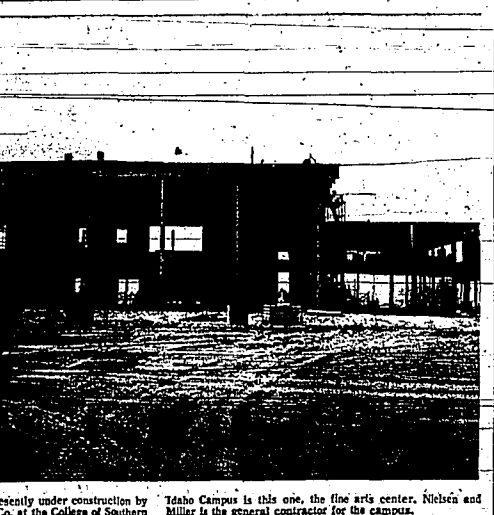
Idaho Campus is this one, the fine arts center, Nelson and Miller is the general contractor for the campus.
