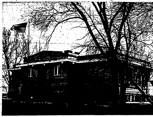
END OF AN ERA for public school instruction in Twin Falls School District No. 411 will come this spring when Union School closes its doors. The school, midway between Fillet and Twin Falls, will no longer offer classes to elementary students.
