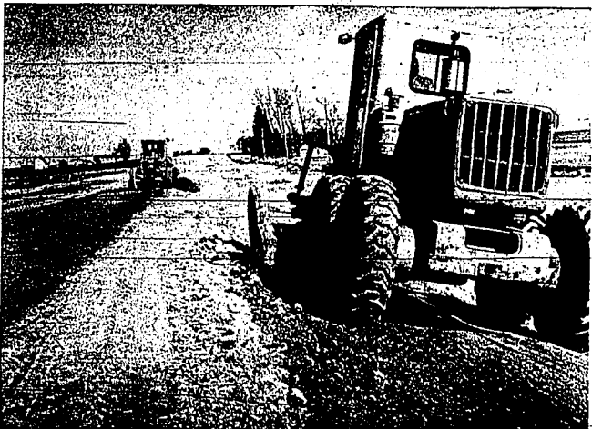
MUCH OF THE ruckus for a completely new section of U.S. Highway 30 between Kimberly and the Hansen bridge is now complete. The 5.2-mile new construction project is expected to be finished by early fall. The complete new route from
