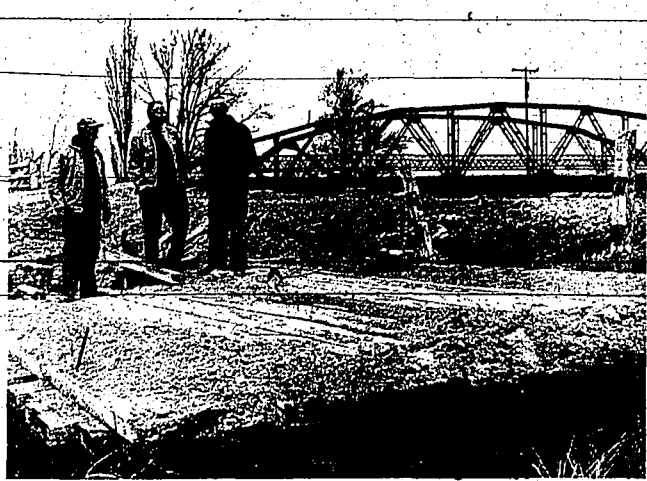
REMAINS OF THE FLOOR of an old canal bridge northeast of the Hansen overpass are surveyed by Murtaugh Highway District Directors Leon Pickett, Joe Saxony and Art Carver. From left, in the background is the district's new steel bridge.
