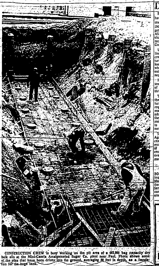
CONSTRUCTION CREW is busy working on the pit area of a 465,000 bag capacity dry bulk silo at the Mini-Cassia Amalgamated Sugar Co. plant near Paul. Photo shows some of the piles that have been driven into the ground, averaging 80 feet in depth, as a foundation for the huge tank.
