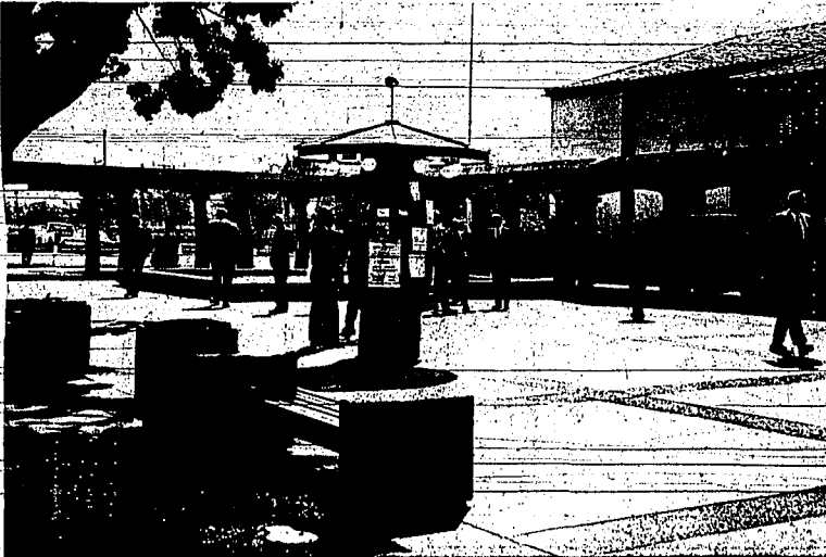
SANTA CLARA'S Post Office is just barely visible in this picture of an interior court in that community's completely rebuilt downtown area. Also noted is a Parliian type bulletin board. Stores border this area.
