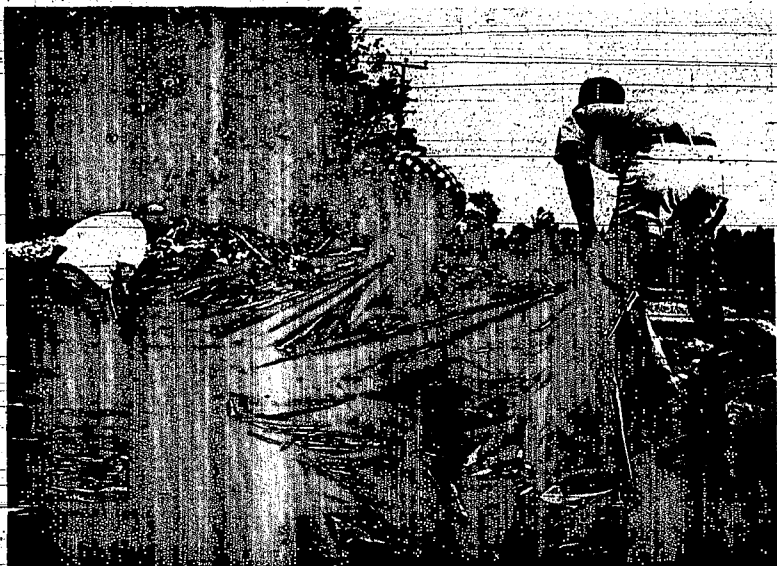
PRECAUTIONARY METHODS, such as sealing wing diversion irrigation dams with plastic as shown here, have been started on the Lemhi River in an effort to break a low water threat and provide sufficient water for anadromous fish passage. This method was successfully employed in 1965 and
