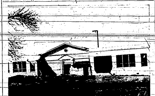
VICTORY SCHOOL, considerably the worse for wear, as it looked a short time ago when we began to tear it down. Less remains today... and shortly no trace will be left of the 1923 structure.
