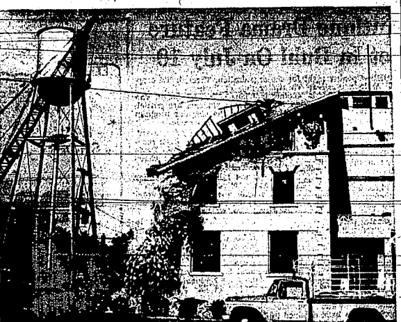
THE OLD LINCOLN INN at Gooding is being demolished. Heavy equipment, owned by Marvin Pierson, is tearing down the old structure and carting away all the rubble. The contract for destruction of the building was awarded to Mr. Pierson for the lowest bid. His bid was $4,000 for the Lincoln Inn and $9,000 for the courthouse. Work of the demolition is to be completed within 40 days.
