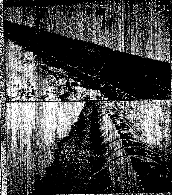
GOOD AND BAD concrete-lined ditches are compared in this photo. The top photo shows a bad ditch with a long crack in the bottom of the ditch, a result of improper placement of material and/or poor installation. The bottom photo shows a good ditch that was installed properly with the proper mixture.
