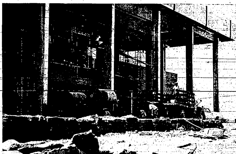
CONSTRUCTION IS PROGRESSING on schedule on the College of Southern Idaho campus. One of three buildings, currently under construction is the Fine Arts Center, shown here from the front. Current work on the huge structure includes the facing of a raised area in front of the building
