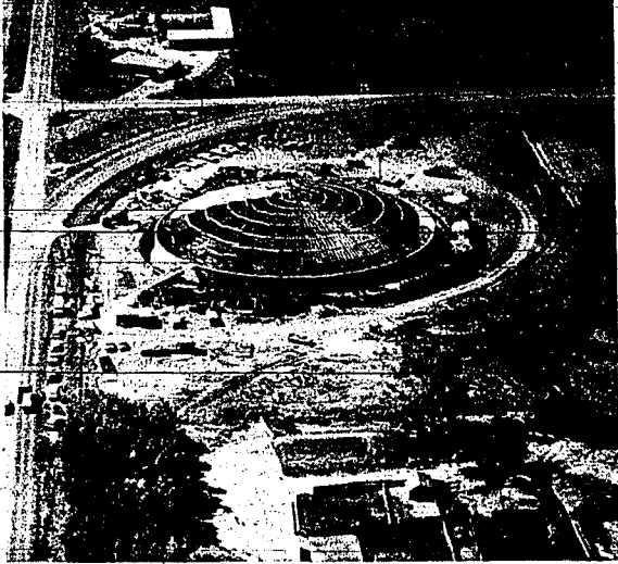
WORK IS PROGRESSING rapidly on the old city water tank south of Twin Falls. This Times-News aerial photo shows the extent of the work. When the tank is covered, it again will be filled with water for use in the city's system. Recently, Blue Lakes water was pumped into the new tank at Harrison Street and Falls Avenue and, after several delays, residents were furnished Blue Lakes water. The high pressure in the system is proof of the worth of the new source of water in the improved and modern water system.
