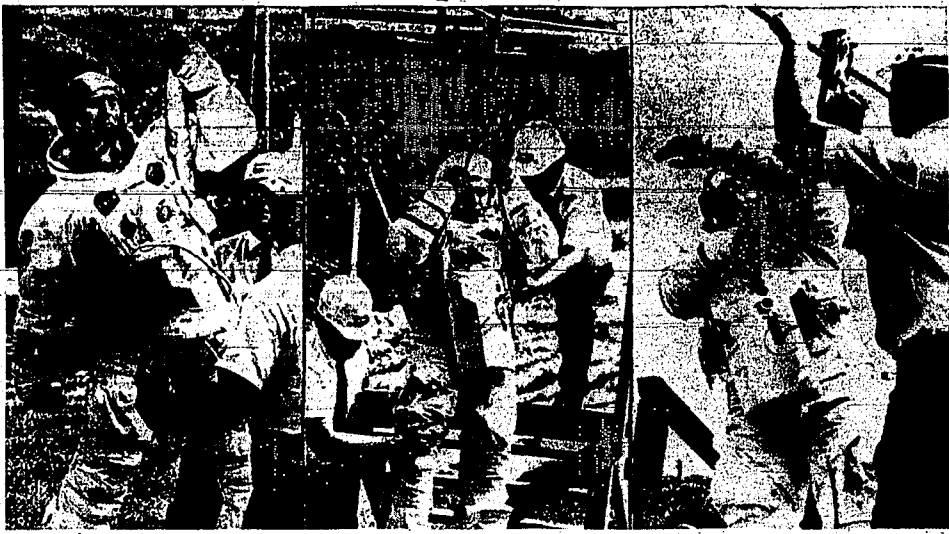
TESTING THE CABLE designed to provide a "slide for life" away from their rocket in the event of an emergency. Apollo 7 astronauts gear up for a realistic runthrough of the procedure. At left, R. Walter Cunningham unspools his harness. In center, Donn F. Elisele gets an assist from technicians, while Walter M. Schirra Jr., on right, slips into his harness for a short run. The device is designed to provide an extra safety factor before launch from the Pad 34 gantry at Cape Kennedy. The Apollo 7 crew is preparing for a fall flight in orbit, with a moon trip still far in the future. (AP wirephoto)
