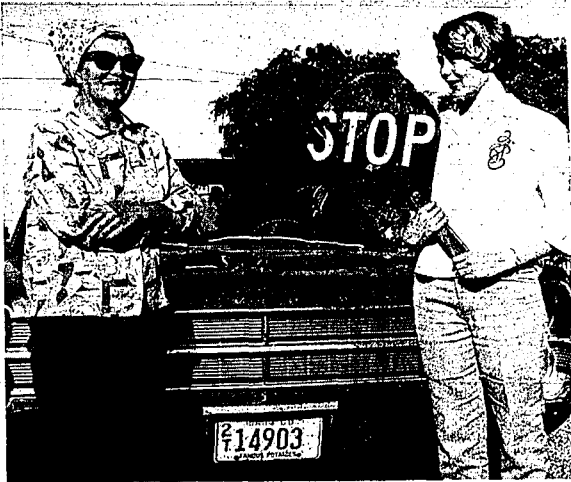
MOTHER AND DAUGHTER. Mrs. Veda B. Drown, left, and Gail Clark, are among the many female "flagmen" working on highway construction projects. Several years ago women flagmen were unusual but today most companies say they use women for this work almost exclusively. Gail is an Idaho State University Student and says this type of work does much more to provide college income than other types of summer work.
