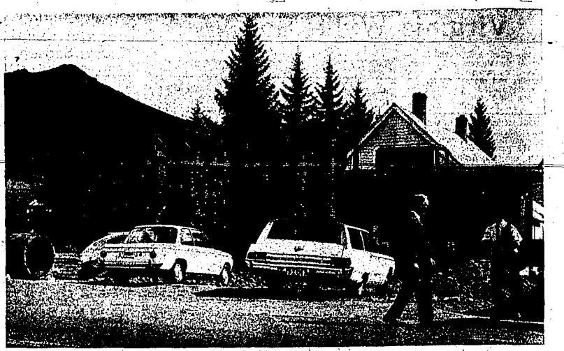
ALTHOUGH THEIR PLANS are not yet definite, a group of Sun Valley men have combined ideas and finances to build what may be one of the most unique restaurants in the Ketchikan area. They have moved ladders from an old water tower to the site and also an old caboose, which will be opened first. Details of the water tower project are not yet complete, according to Ned Bell, insurance man; Bob Wright, Sun Valley advertising man; Buhl Ames, night watchman; Paul McKinnon, captain of Challenger Inn bowling, and Gordon Butterfield, ski instructor, who is dubbed the "idea man."
