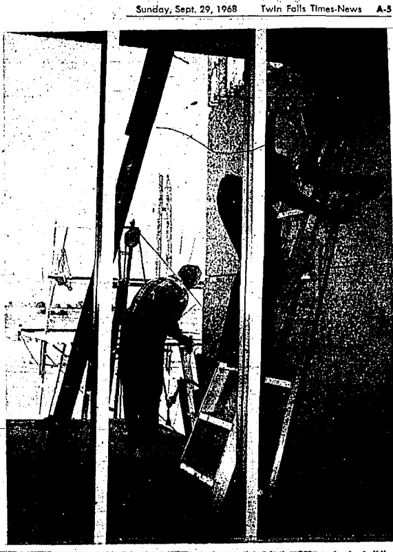
PRE-CAST DECORATIVE SLABS on an exterior portion of the CSI academic building receives some finishing touches from workmen on the project. The men are applying a caulking compound to grooves between the slabs. The photograph was taken from a second-floor corner lobby, with the CSI tower visible in the background.
