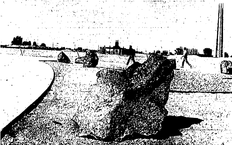
INITIAL LANDSCAPING SHOWS a preview of things to come as workers place large rocks, gravel patterns, sunken gardens and other decorative touches throughout the campus and around buildings. Accents in the landscaping, seen in the background, include the college tower at right and Oriental design which covers one of the small utility buildings.
