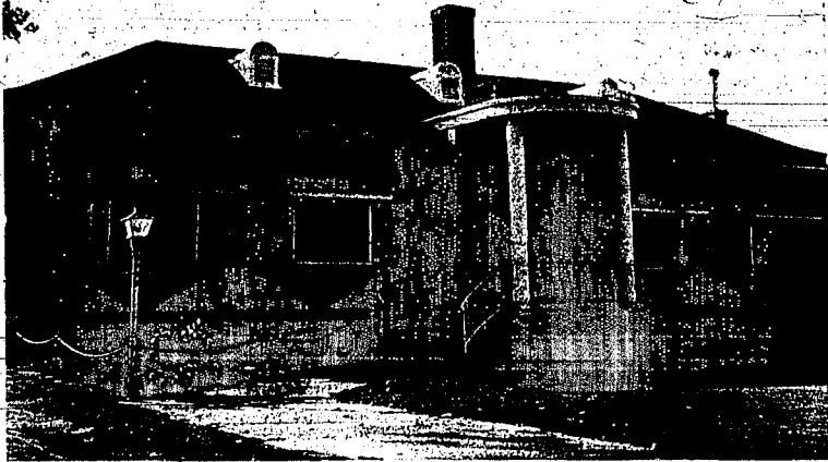
CONVERTED FROM a two-room single story red brick schoolhouse to be a "show place" home is the above home of Mr. and Mrs. W. E. Munger and their two children. Once the Shamrock school, the building was sold by the school
