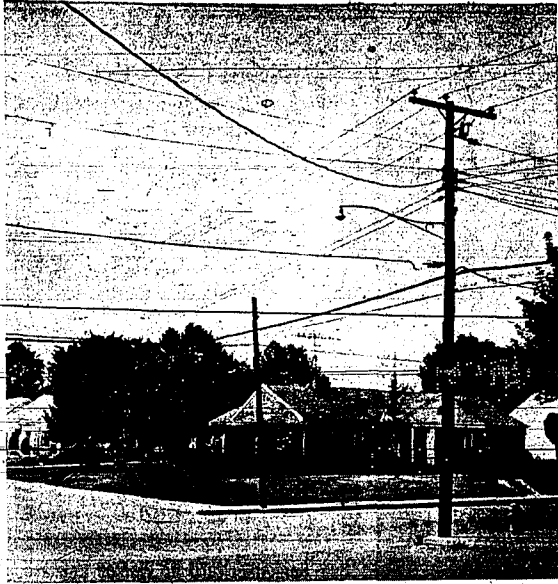
SCENES LIKE THIS ONE will someday be part of the past, say members of the U. S. Independent Telephone Association. All major utility companies as well as residential and industrial developers and in most cases municipalities are working toward underground utility lines. Not only do officials feel there is much to be gained aesthetically but overall maintenance costs are less on underground installations.
