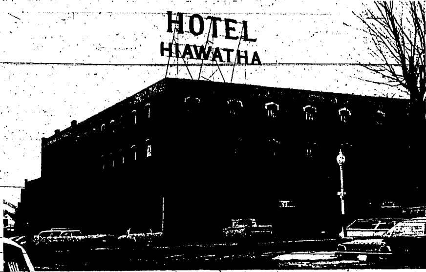
PIIONEER HIAWATHA HOTEL that dates back to the turn of the century has just undergone some major changes. The exterior of the building is much the same as it was more than 65 years ago, but on the inside things are different. Located in Halley, the hotel was built during the mining era and has just been renovated to meet the demands of the present Wood
