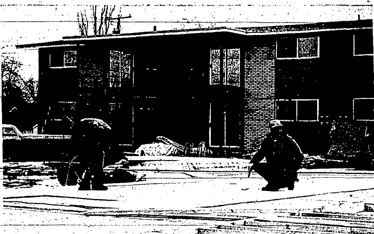
THE TOWNCREST MANOR near the Twin Falls city hall is taking shape. Workmen are putting a floor down here while the apartments-of-the-manor loom in the background. The apartments are being built by Wills, Inc. They will rent for $102 a month, all utilities including heat will be provided.
