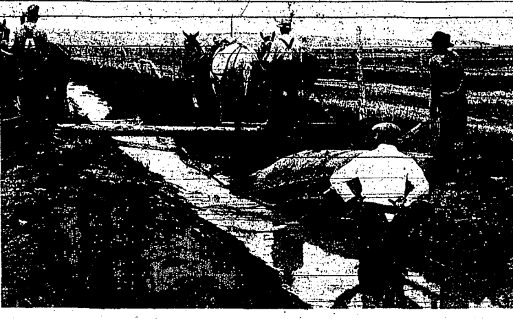
Early day ditching operation on canal system.
