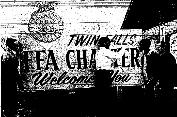
WELCOMING SIGN is being erected on the north edge of Twin Falls by the Twin Falls FFA Chapter in preparation for the State FFA Convention next week. Over 700 FFA members from throughout Idaho are expected here for the three-day confab. Erecting the sign on Blue Lakes Boulevard North are
