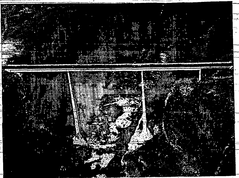
THE NEW HANSEN BRIDGE WAS COMPLETED IN 1966 under the direction of the Idaho Department of Highways. It replaced the 47-year-old Hansen Suspension Bridge, often called the "Swinging Bridge." Built before the Perrine Memorial Bridge, the old Hansen span was begun in 1917 and dedicated in 1918. The old bridge, built for wagon traffic, was suspended between two towers on each side of the canyon. The strong wind conditions which sometimes prevailed through the canyon gave rise to the bridge's nickname, "Swinging Bridge." The new bridge can withstand winds of up to 100 miles per hour according to engineering claims, and offers motorists from Twin Falls and Kimberly a direct route to Interstate 80N between Burley and Jerome. (Idaho Dept. of Highways photo)
