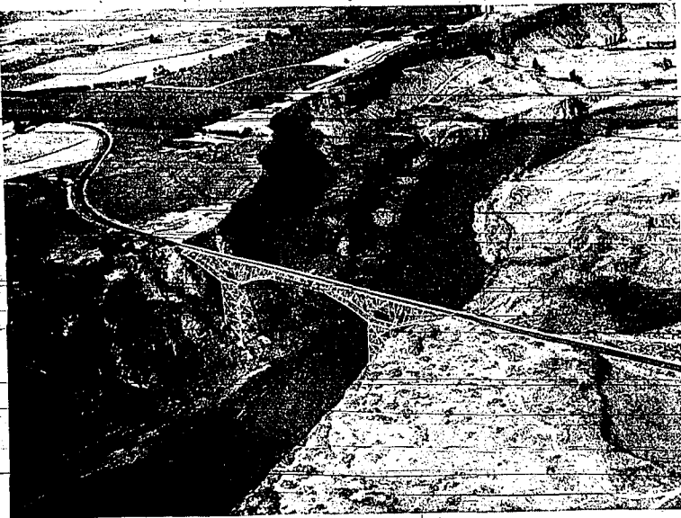
PURCHASED IN 1913 FOR LESS than $500,000, the Perrine Memorial Bridge is now maintained by the Idaho Department of Highways. In the past year the road surface of the bridge received a new sealcoat and every 15 or 20 years the bridge is repainted. Currently an inspection of the bridge is underway. The Southern Idaho landmark was built in 1927 by the Puget Sound Bridge and Dredge Co. When completed the nationwide interstate highway system will be a 41,000-mile network of high speed, high capacity, controlled-access roads. (Idaho Dept. of Highways photo)
