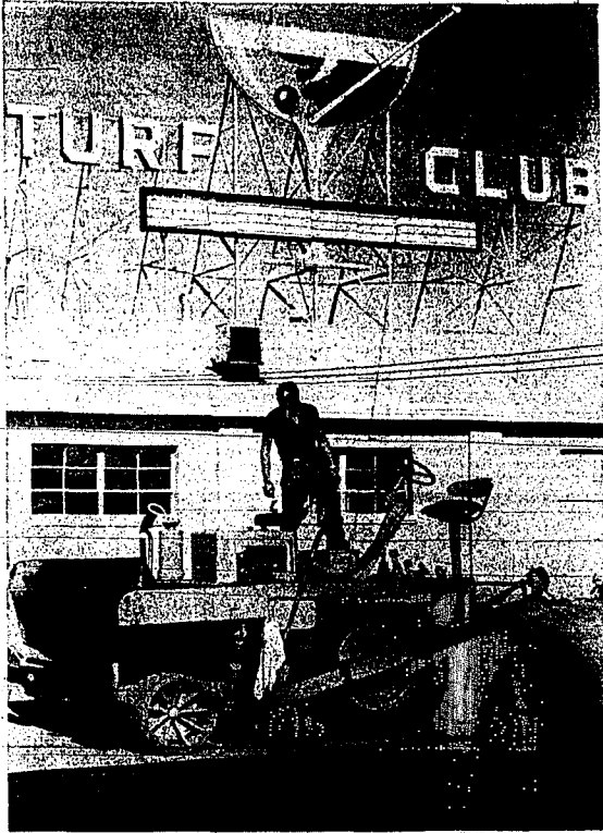
PAVING THE TURF Club parking lot is the crew from Beymer Paving, Inc., Twin Falls. This is the first job for the new firm, which is owned and operated by C. B. Beymer. Mr. Beymer said the company will specialize in small paving, grading, graveling and stripping jobs. The Turf Club is expected to open to the public about May 15. Leo Soran, owner of the club, said banquets are being scheduled from May 1.
