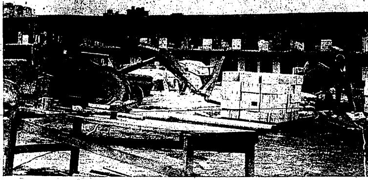
CONSTRUCTION WORK IS well under way on a new addition to the Cactus Pete's Motel, Jackpot. Contractor for the 50-unit installation is Nelson and Miller Construction Co., Twin Falls. It is anticipated that the units will be ready for occupancy by the middle of June.
