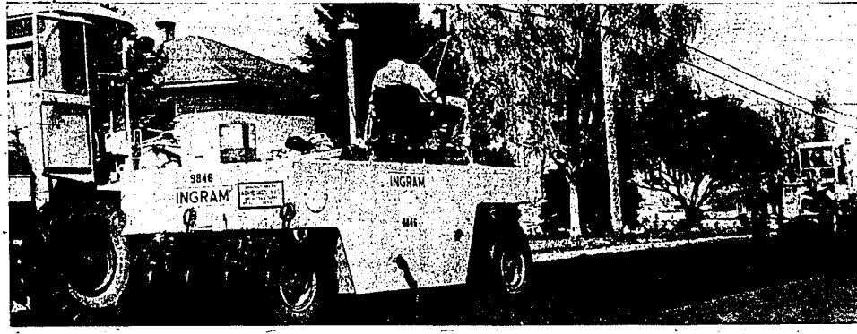
STATE HIGHWAY EQUIPMENT and crews are "patching" Highway 30 west of Twin Falls. Breakup of the upper roadway has been so complete-patching work resembles a new surface. When the asphalt work is complete, contractor Cary Nelson, Logan, Utah, will move into the area to put a plant mix overlay on the entire roadway. Similar work is
