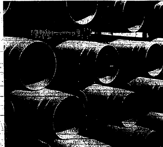
TRANSITE PIPE IS USED in the new Hansen sewer project. It is reportedly better than concrete and is easier to use. Connections prevent tree roots from getting into lines which constitutes a major problem in sewer maintenance.
