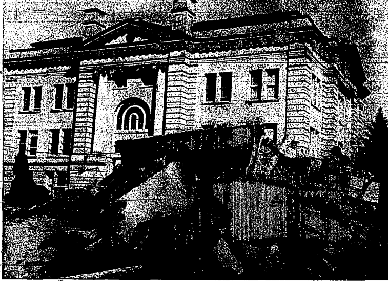
PARKING LOT AT Twin Falls County Building is being "remodeled." The work is expected to take several weeks after which the available parking area will be greatly enlarged. Here a piece of heavy equipment removes section of a former sidewalk. County officials urged motorists to not park on the area until completed. This caused some citizens to raise an eyebrow and wonder just who would attempt to park there under the circumstances.
