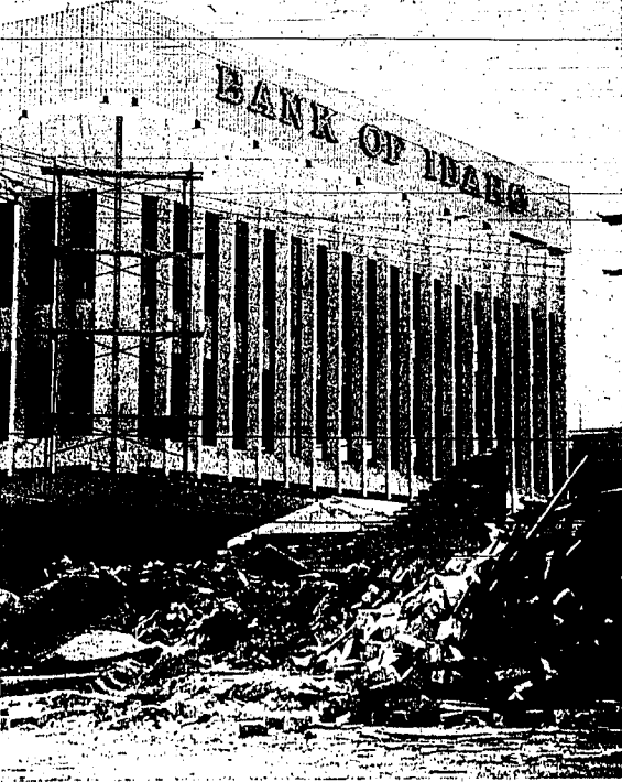
WHERE THERE IS NEW construction there is bound to be new destruction, and this picture shows both. The new Bank of Idaho building is seen in the background and the rubble of the old Dean Motor Co. building is in the foreground, minutes after the building was torn to the ground. The Dean Motor Co. property is being converted into a parking lot. The new bank is expected to open in a month and workmen are pressing hard to meet the deadline.
